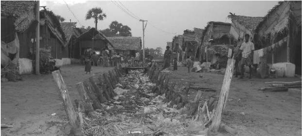
In this temporary settlement unit, although the streets are kept clean, garbage is thrown into gutters that are meant to drain out rainwater. Water collected here cannot flow easily into designated sewers.
