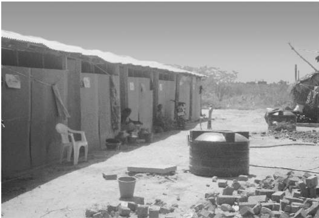
Tin sheets are conductors of heat. By extending the roof towards the entrance of the house, a provision for shade is created.
