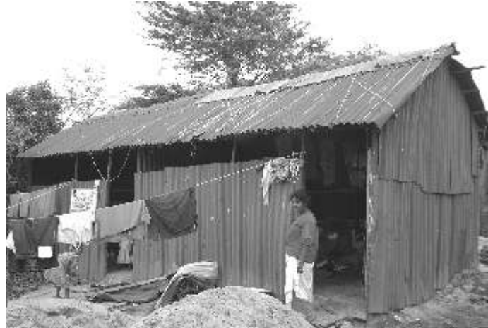
The gap between the roof and the wall of the shelter ventilates the shelter and brings in natural light during the day
