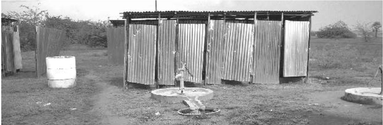
The path to the toilets is stagnant with water. An appropriate solution is to raise the plinth level of the toilet and also to pipe the used water into septic tanks located behind the toilets.
