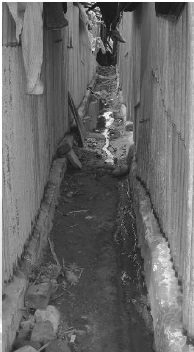
The path to the toilets is stagnant with water. An appropriate solution is to raise the plinth level of the toilet and also to pipe the used water into septic tanks located behind the toilets.
