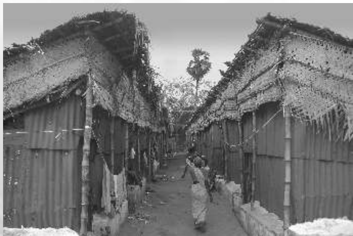
Thatch used both for the roofs and to cover the gap provides some amount of cooling. Nevertheless there is a risk of fire, the prevention of which requires taking precautionary measures.
