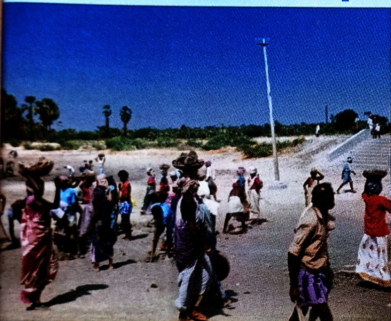
Involvement of people in rehabilitation work
