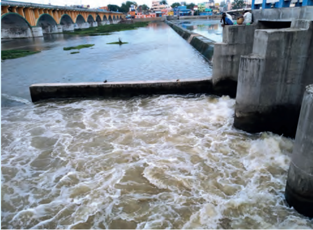
Kalpalam Check dam
