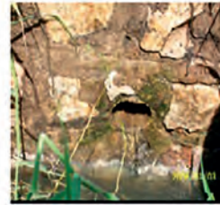
(c) Effluent comes out of FDS
