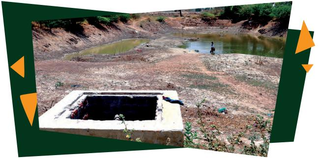
outlet structure such as waste weirs, conduits to release the surplus water. The surplus water either feeds neighbouring tanks or connects with the storm water drainage.
