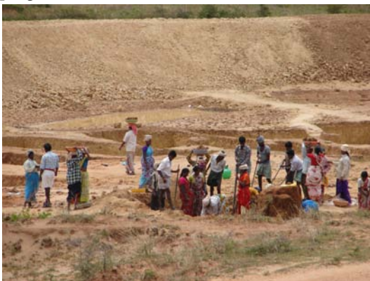
Desilting and rehabilitating the tank: A work in progress
