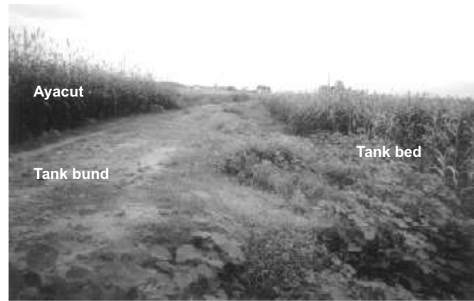
A typical encroachment in tanks
